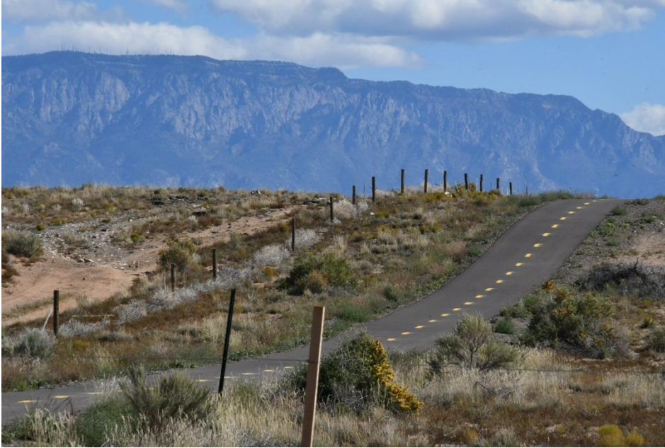
The newly repaved Paseo de la Mesa trail heading east from the Ruth Eisenberg Trailhead. Photo by Bill Pentler
